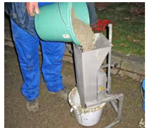
Dosometer for verification of fibre dosage in fresh concrete
