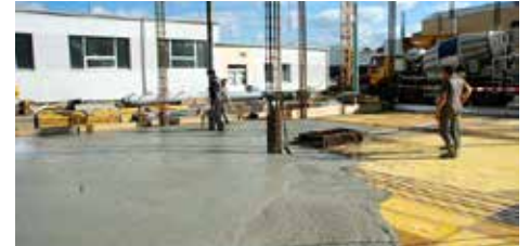
Installation of a TAB-Slab® with 100 kg/m 3 dosage rate
