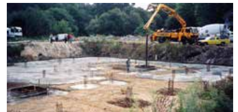
Installation of a pile supported TAB-Raft® with 65 kg/m 3 dosage rate
