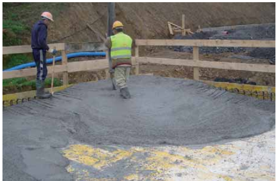
Figure 1: Placing a TAB-Slab concrete at LKS site in Mondragon (Spain).
