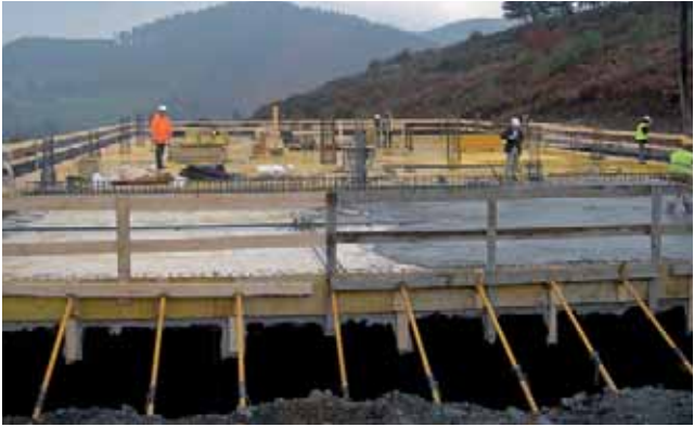
Figure 9: LKS office building with TAB-Slab pouring in progress; APC reinforcement is also visible.
