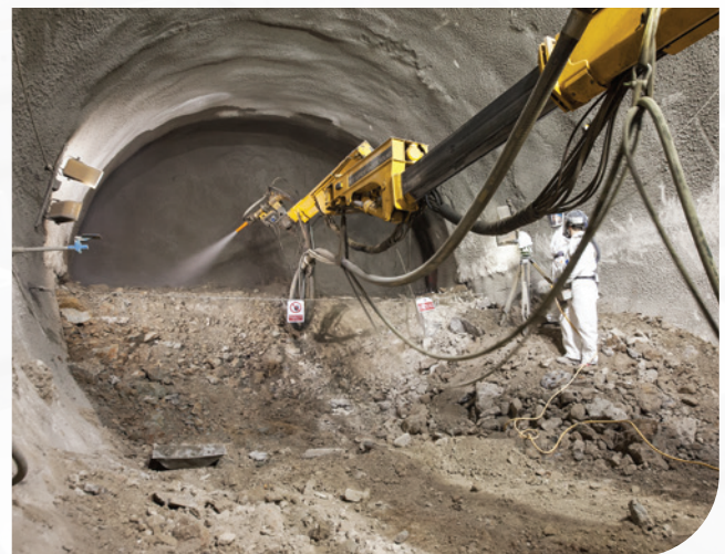
Shotcrete works at Crossrail, London © Crossrail Ltd.
