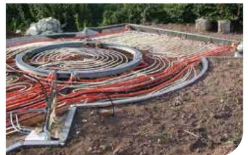
Raft with integrated floor heating, Bendorf (D)
