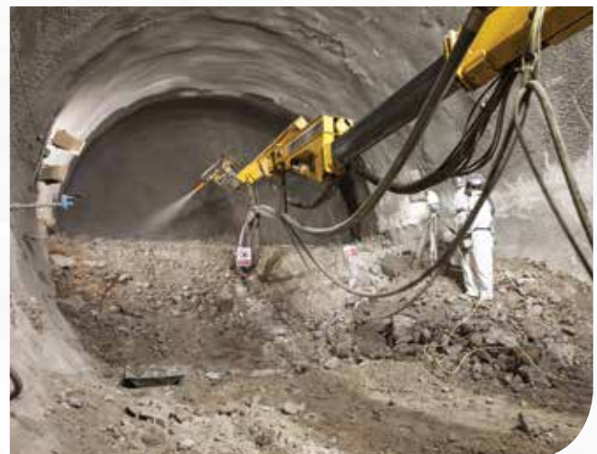
Shotcrete works at Crossrail, London © Crossrail Ltd.
