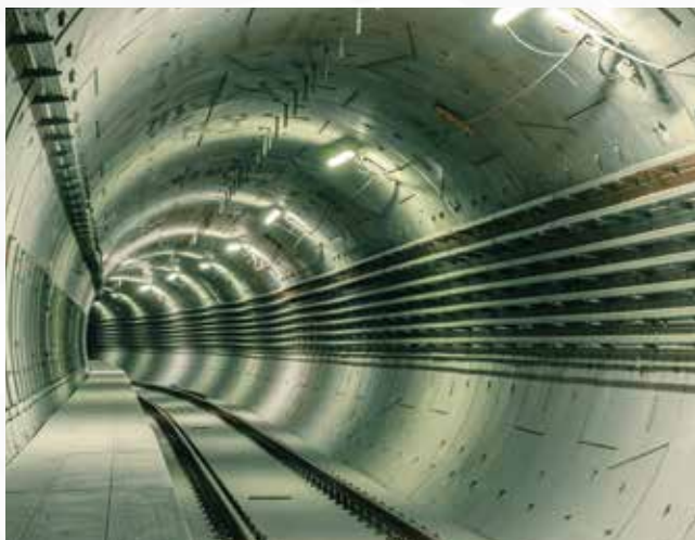
Installation of fibre reinforced tunnel segments, Doha Metro, Qatar.
